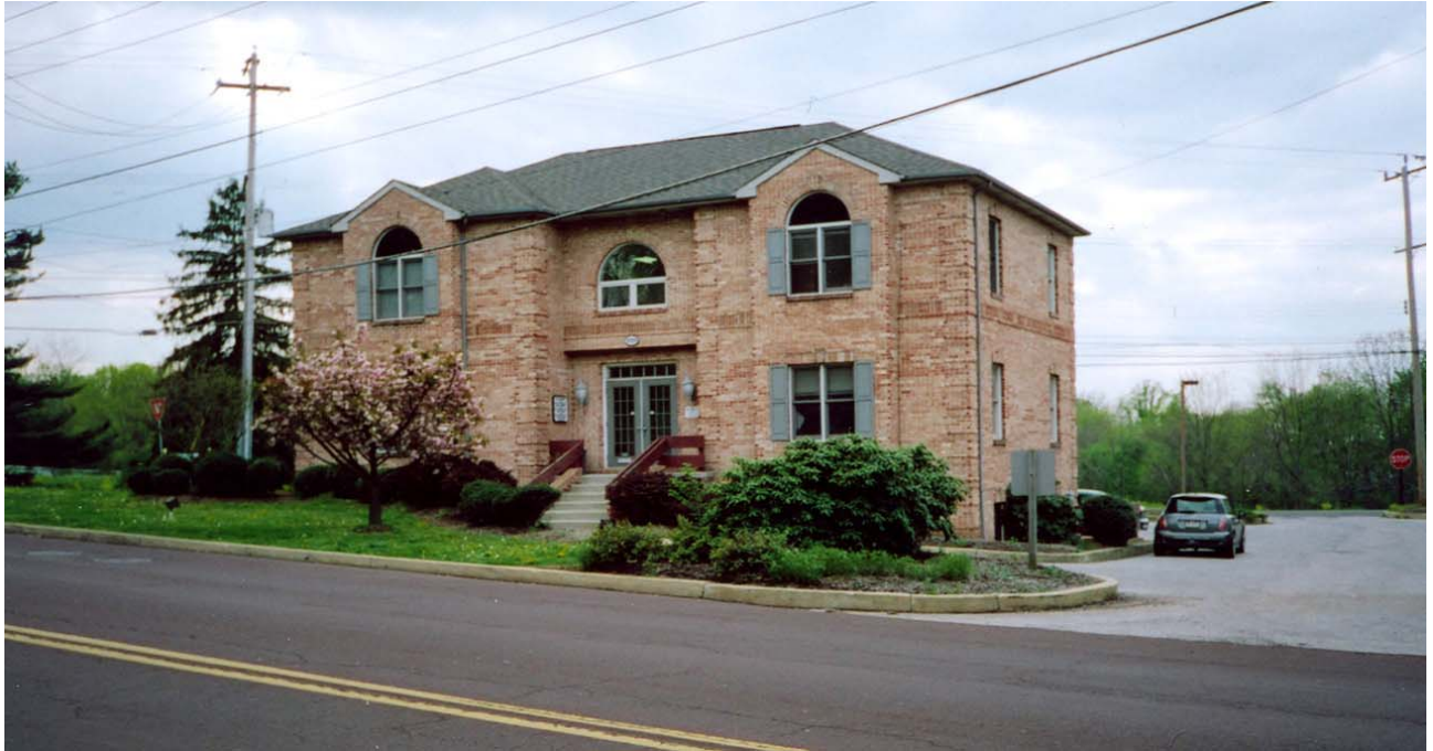
Above is a current picture of the building at Broad and Allentown Rd where the first Lansdale office was located. Below is a picture from the Prescription taken on opening day.
